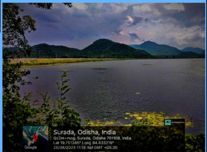
Photograph No: 4.4 Surada Dam
